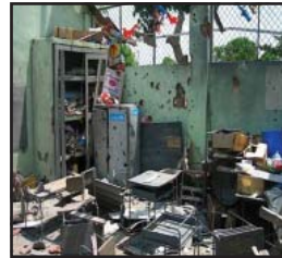
Classroom devastated as a result of aerial bombing by SLAF
