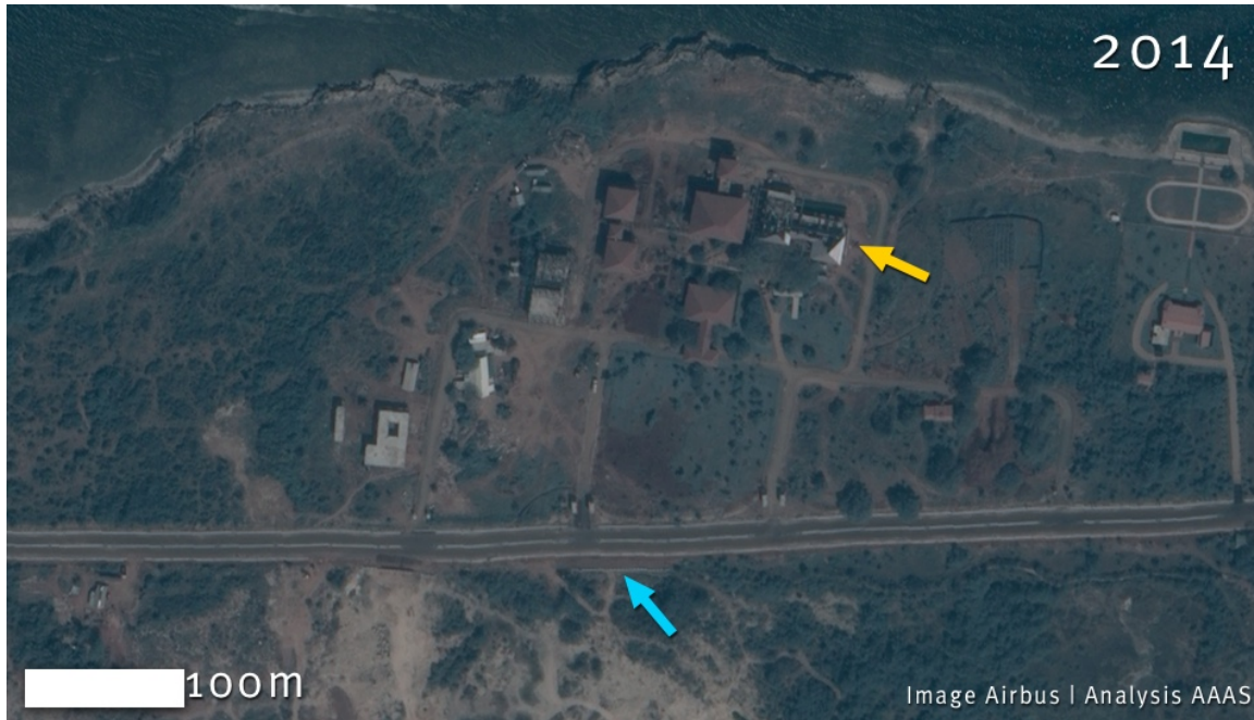
At a site near Thalsevana Holiday Resort, only two buildings are visible in 2009 (red arrows, top image). In 2011, an additional building is under constructions (purple arrow, middle image). Finally, between 2011 and 2014, this site changed dramatically (bottom image). The road running east-west below the complex has been expanded substantially (blue arrow), and numerous buildings have been added to the site, including one building under construction that has a footprint of 1,600m 2 (yellow arrow). Top and middle images: DigitalGlobe| Bottom Image: Airbus Defense and Space | Analysis AAAS. Location: 9.815N, 80.021E.
