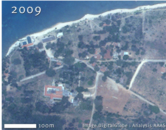
Figure 8: Additional large development along HSZ coast
