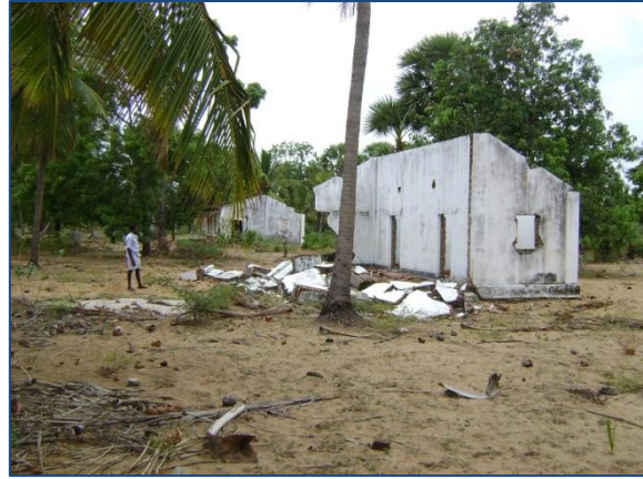
Damage from the tsunami in Sri Lanka (Danesh Jayatilaka, January 2011)
