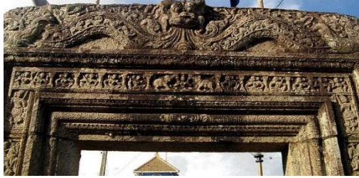
Stone gateway of Tenavarai temple destroyed by the Portuguese
