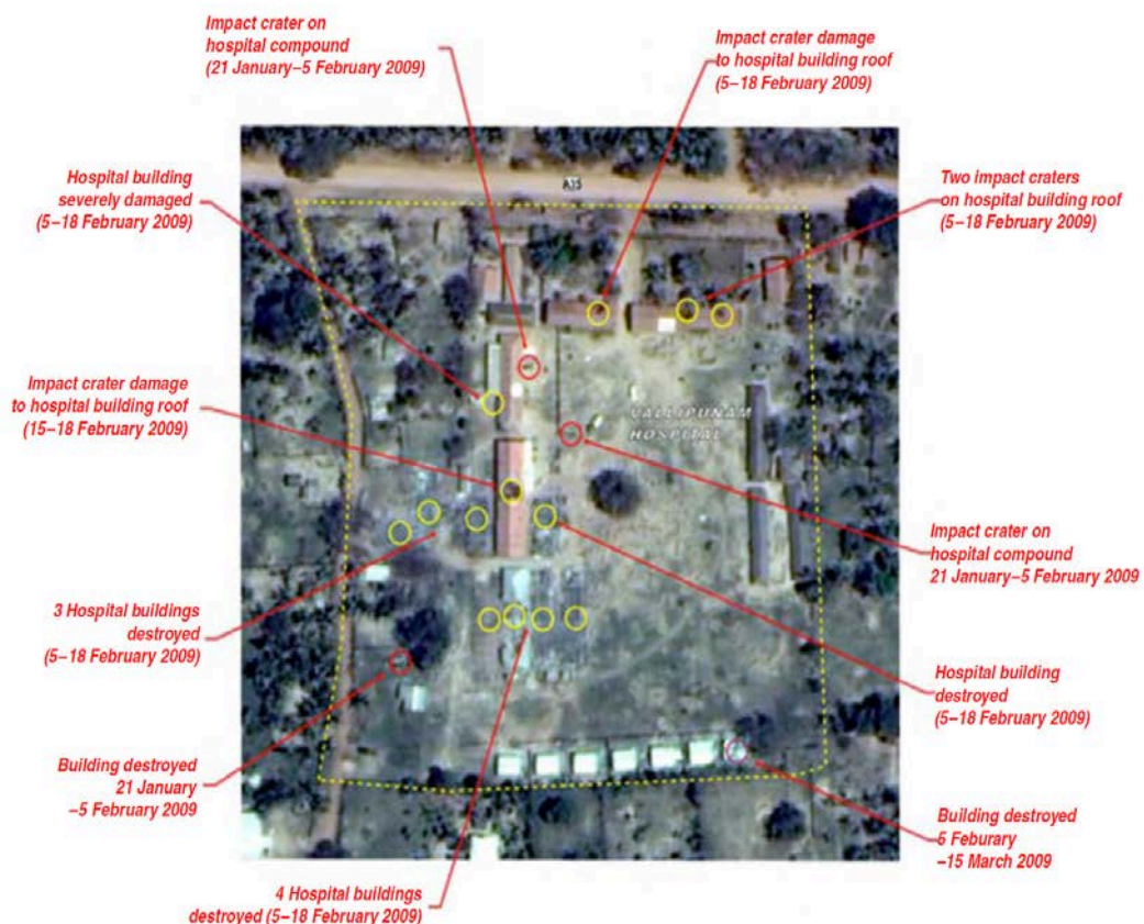
Figure 7: Satellite-based damage assessment for Vallipunam hospital, Sri Lanka (UNITAR/UNOSAT).
